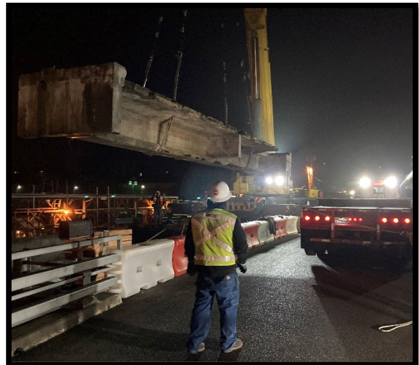
Removal of deteriorating girders, Anacortes Ferry
