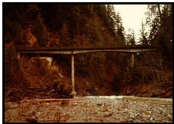
Upper Finney Creek Bridge
