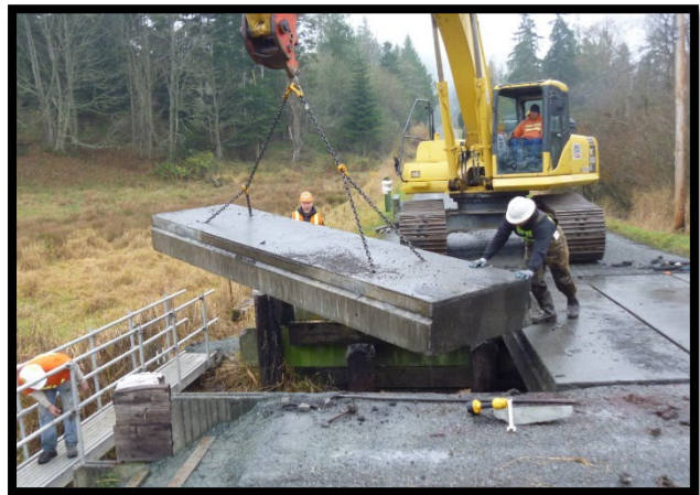
Campbell Lake Outlet receiving new timber cap, 2013
