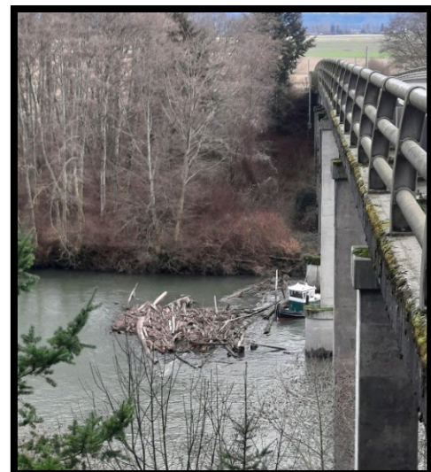
North Fork Bridge, debris removal
