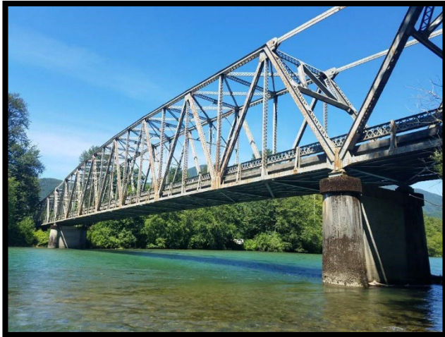
Marblemount Bridge – Skagit River
