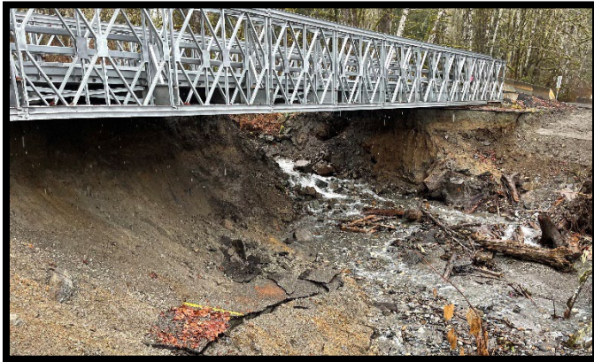
Concrete-Sauk Valley at North Osterman
