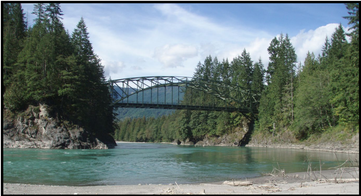
Dalles Bridge near Concrete (Concrete-Sauk Valley Road)
