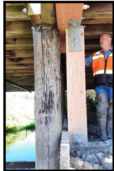
Old 99 at Thomas Cr, temp shoring
