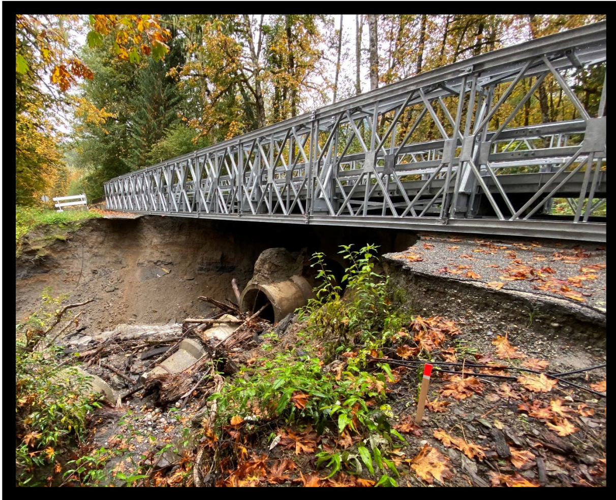
“Concrete-Sauk Valley Temporary Bridge”
