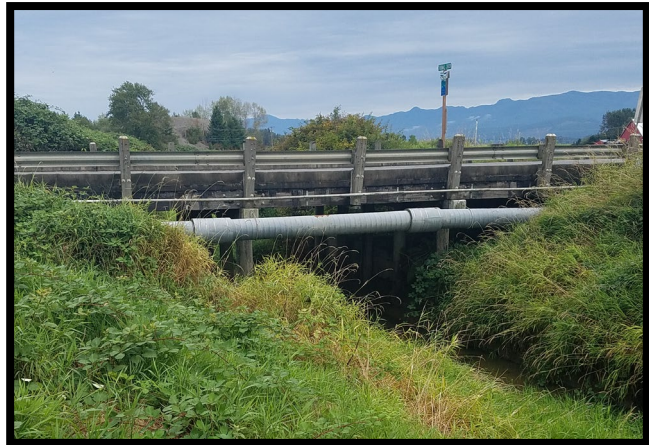
Thomas Creek Bridge – Old Hwy 99 N.
